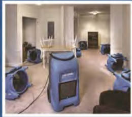
Structural Drying
